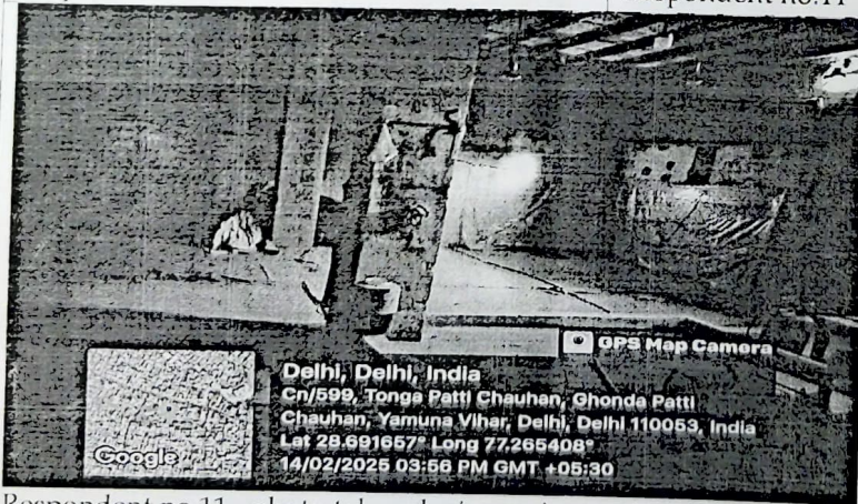
Respondent no.11 , photo taken during re-inspection
