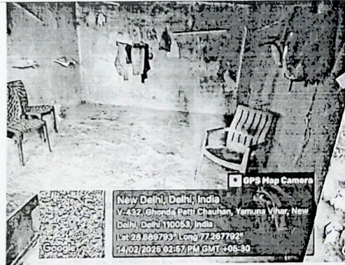
Respondent no.35, photo taken during re-inspection
